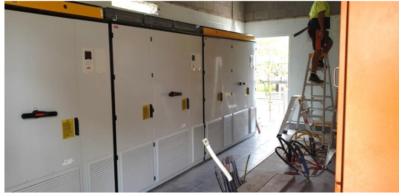
New ABB AC880-37 Drives being retrofitted into the existing switch house.
