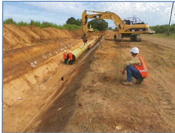
Figure 9: Capital Works: pipeline replacement
