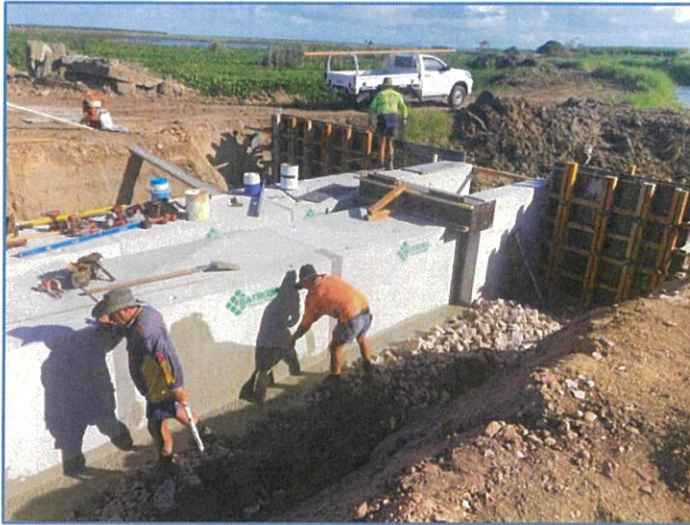
Figure 8: Installing new culverts at McAllister Road
