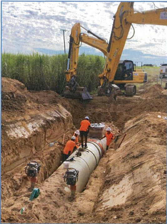
Figure 6 Capital works infrastructure project: Construction of the replacement McDowell Pipeline.
