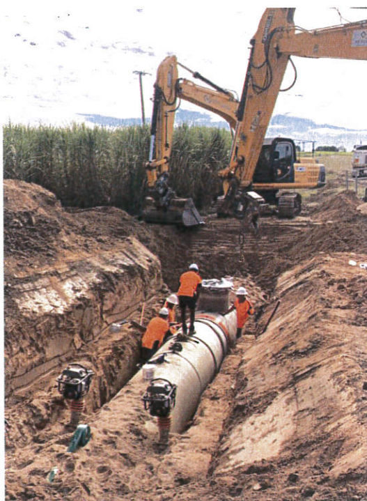
Capital works infrastructure project: Construction of the replacement McDowell Pipeline.
