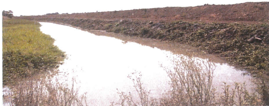
Water Distribution Channel
