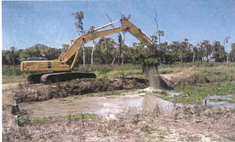
Channel Cleaning Using Mechanical Methods
