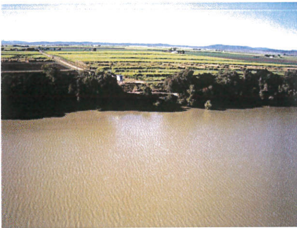
McDowells Pump station on the Burdekin River
