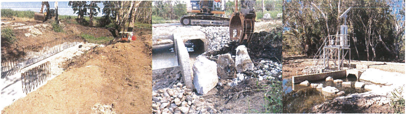
Capital works infrastructure project: Construction of the Saltwater Creek automated water control gates, channel crossing and fish ladder.
