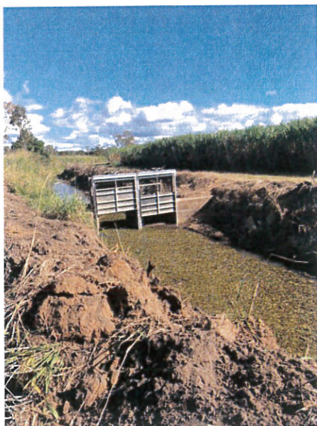
Capital works infrastructure project: Construction of the Saltwater Creek automated water control gates, channel crossing and fish ladder.
