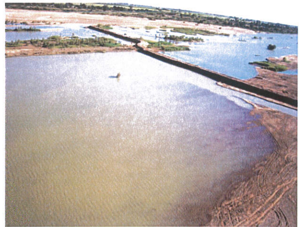
Temporary Sand Diversion Structure located on the Burdekin River
