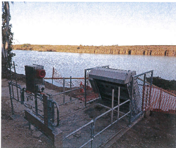
Capital works infrastructure project: Klondyke Lilliesmere automated weed screen and variable speed drive.
