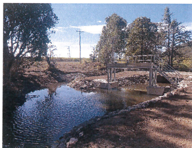
Capital works infrastructure project: Inkerman Station Road automated water control gate and fish ladder
