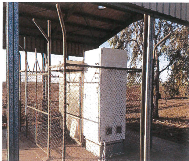
Capital works infrastructure project: Klondyke Lilliesmere automated weed screen and variable speed drive.
