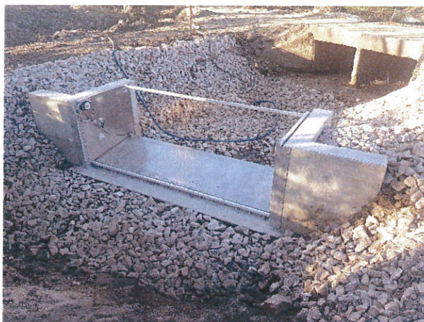
Capital works infrastructure project: Inkerman Station Road automated water control gate and fish ladder
