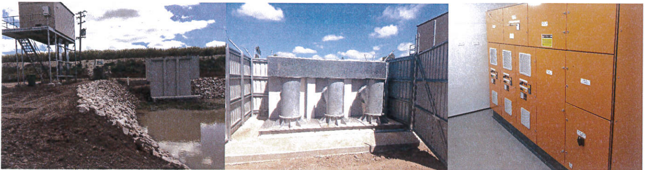
Capital works infrastructure project: Lilliesmere pump station and control room upgrade.
