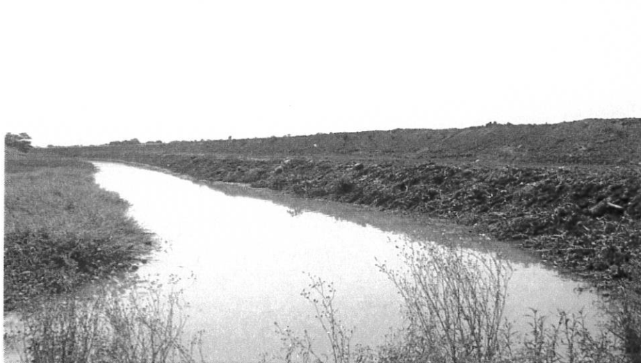
Water Distribution Channel
