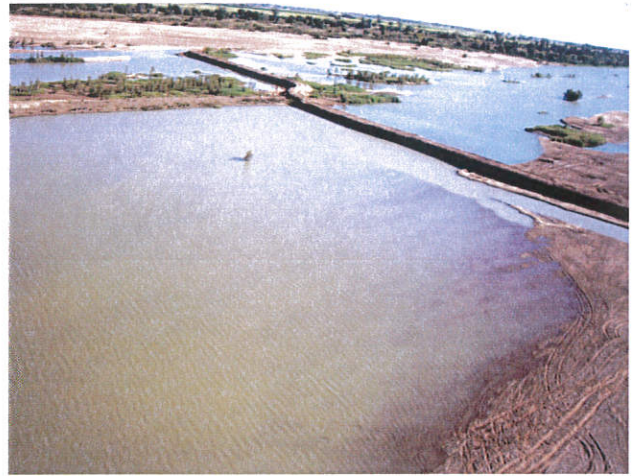
Sand dam located on the Burdekin River
