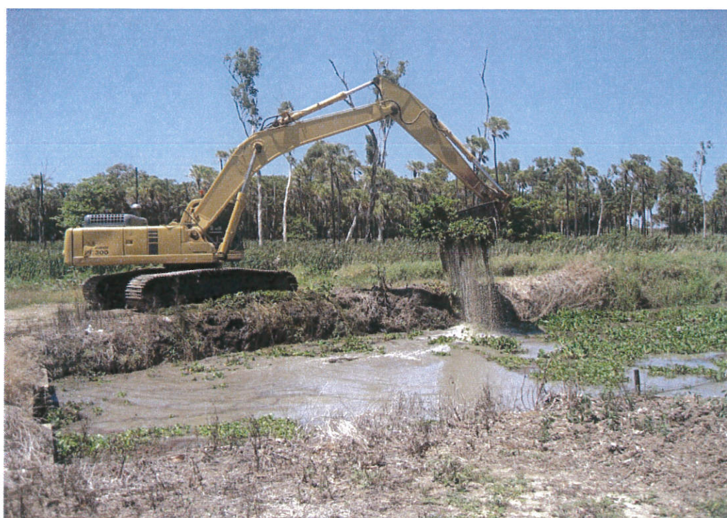
Channel Cleaning Using Mechanical Methods
