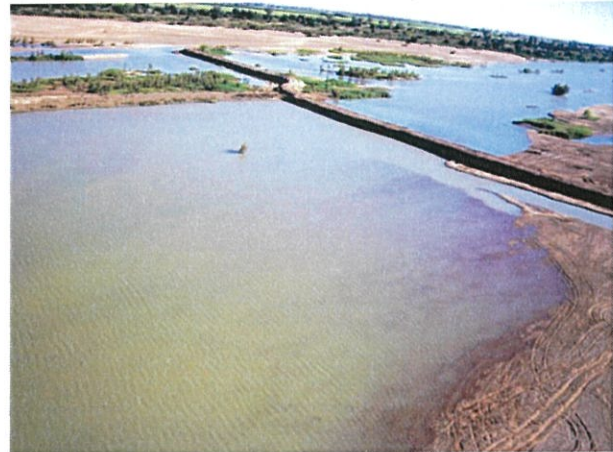
Temporary Sand Diversion Structure located on the Burdekin River
