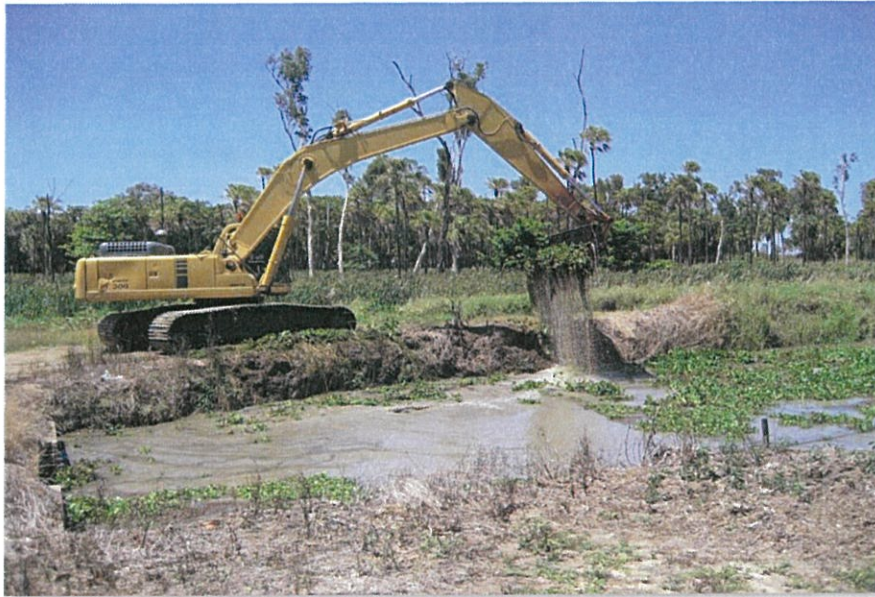
Channel Cleaning Using Mechanical Methods
