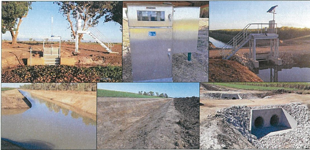
Capital works infrastructure project: Construction of the Red Lily automated water control gates, pump VSD, channel augmentation and channel crossing.
