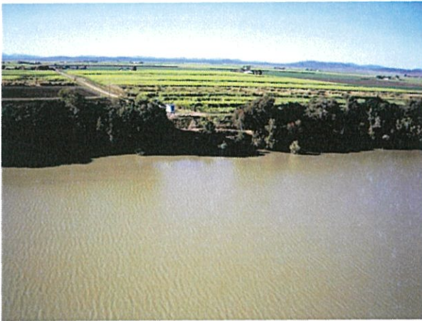
McDowells Pump station on the Burdekin River
