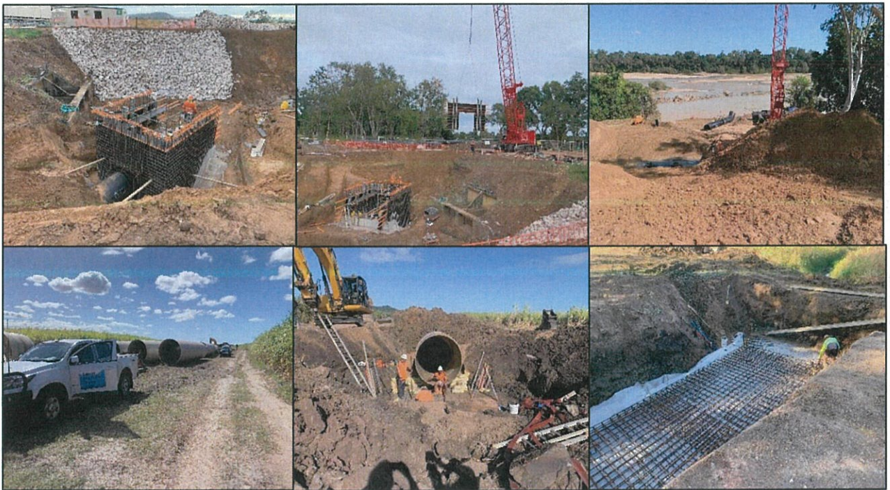
Figure 7: Capital works infrastructure project: Construction of the Warrens Gully Pump Station outlet structure, new inverted siphon and Barry Road culvert crossing.
