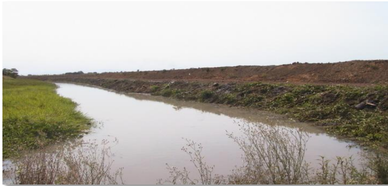
Figure 1: Water Distribution Channel
