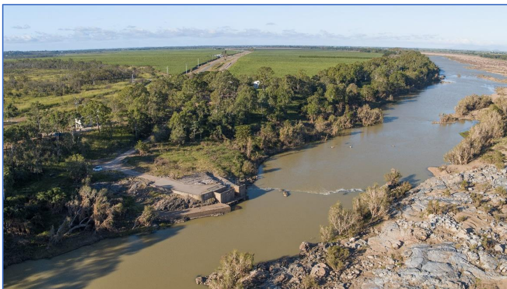
Figure 5: The Rocks Pumpstation on the Burdekin River
