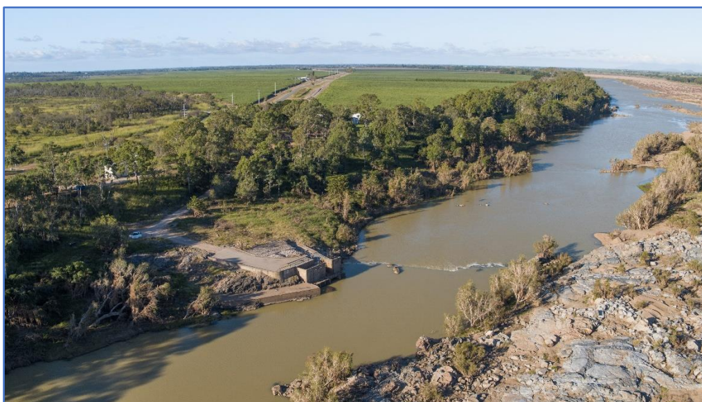
Figure 5: The Rocks Pumpstation on the Burdekin River
